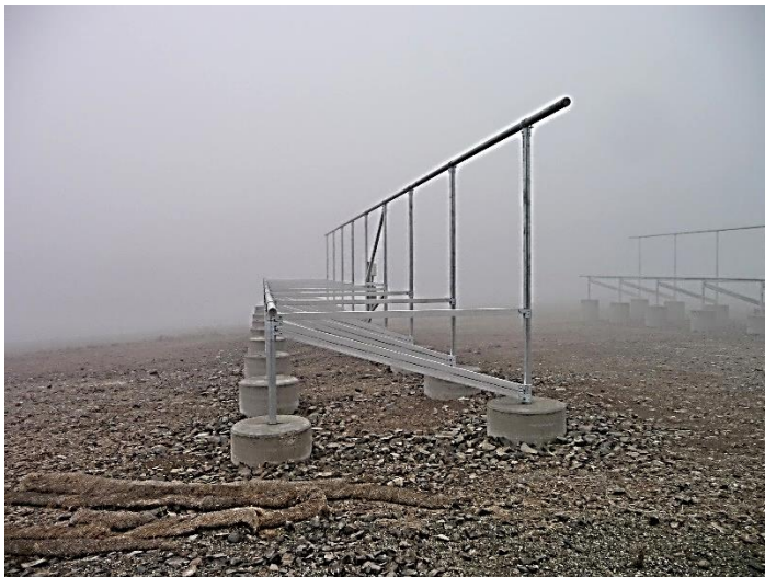
Support structure ready for panel installation
