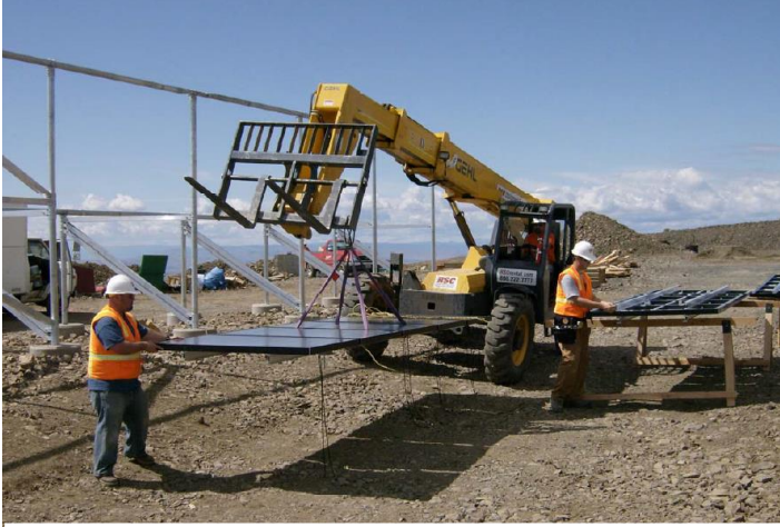
Setting and connecting panels onto the support structure
