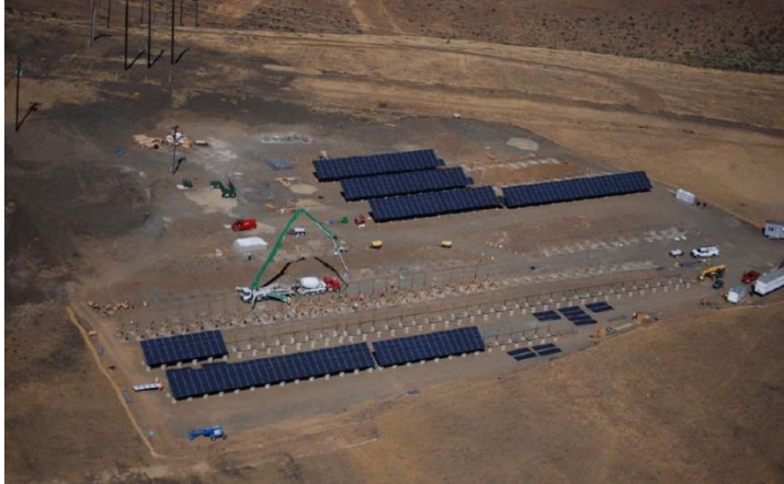
An aerial view of the 450-kW array under construction.
