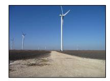
This photo is a wind turbine with a hub height of 67 m (220 ft) and a three-blade rotor with a diameter of 80 m (260 ft). The maximum capacity is 1.8 MW for this specific turbine. Installed in 2007, more recent **onshore wind turbines** have hub heights of 100 m or more, substantially larger rotors, and capacities up to 5 MW or more per turbine.
