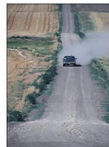
Dust. The amount of dust generated by gravel or unpaved road is a function of: • Silt content of the surface material • Weight of the vehicles using the road • Gravel mixture content (%), and • Vehicle speed.
