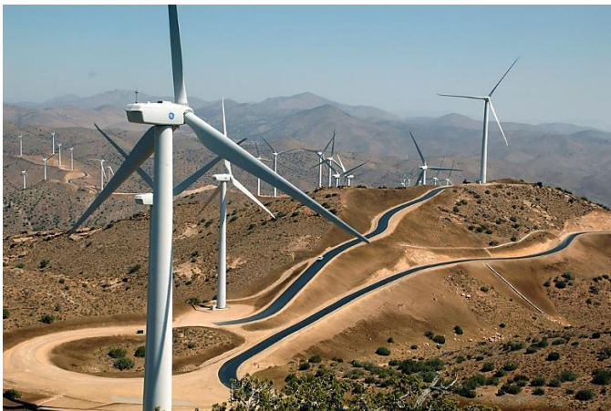
These are the types of roads of interest in this Brief. Photo courtesy of Kiewit Wind.
