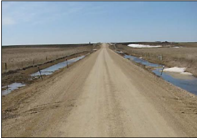
A gravel surface road in good condition. The primary load supporting portion of the structure is crushed stone.
