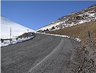
A vertical curve on a mountain road. Note the cut section.
