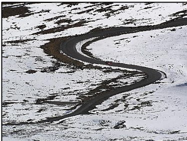
A combination of vertical and horizontal roads. The horizontal curves minimize the vertical curves which reduces cut and fill.
